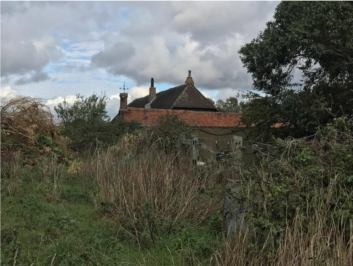
Plate 9 West Tilbury Hall from the scheduled earthworks
