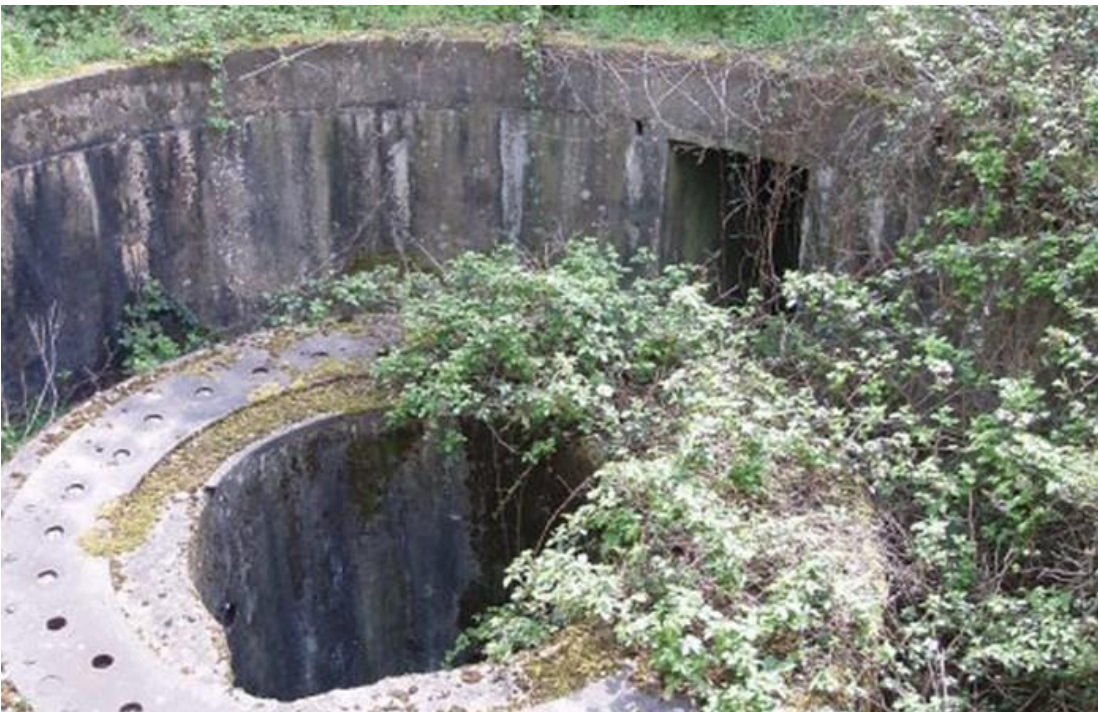
Plate 6 Remains of HAA battery at Bowater Farm
